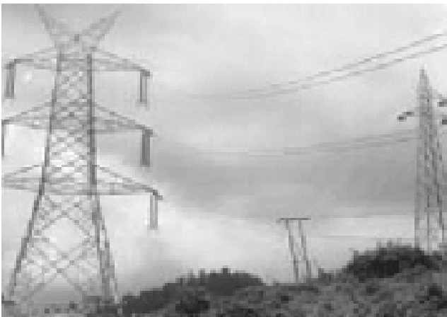
Improper alignment of transmission lines can cause breaks in habitat connectivity
